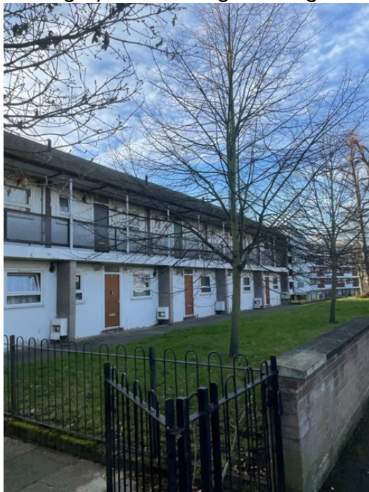
Photograph of existing Seavington House
